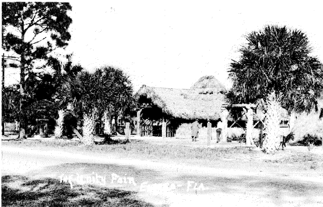
illustration 4.81 Rustic Tea Garden - Exhibition Hall seen from southwest (Koreshan State Historic Site)
