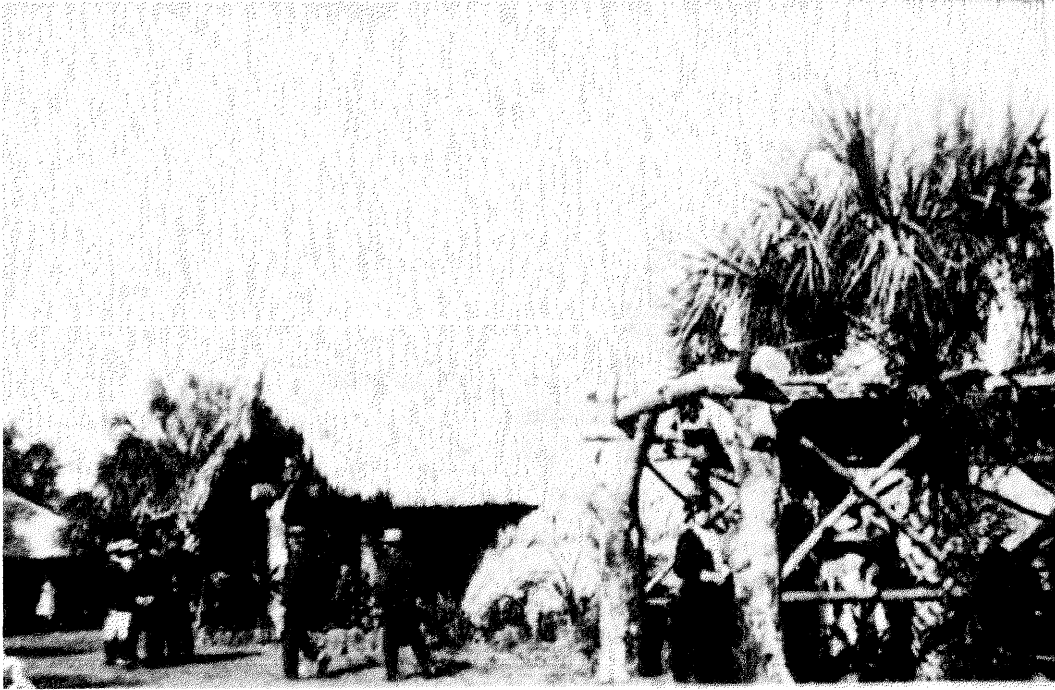
illustration 4.84 Rustic Trellis Garden seen from southwest (Koreshan Unity Foundation) In the right foreground of this photograph, the rustic trellis is seen, with the Exhibition Hall in the background. The logs used as front vertical supports are very thick in comparison to the figure at the right; there are several smaller sizes of rustic members
