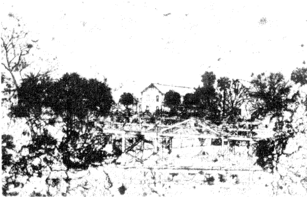
illustration 4.10 Edith Campbell drawing of the bridge over the Estero River, believed to date to the late 1890's (Herbert-Reeves, p. 54)
