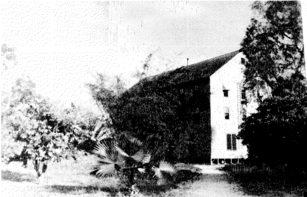
illustration 4.59 Dining Hall and grounds to north (Koreshan Unity Foundation) In this view of the Dining Hall from the north, plantings of a variety of trees, bamboo and palm are seen.
