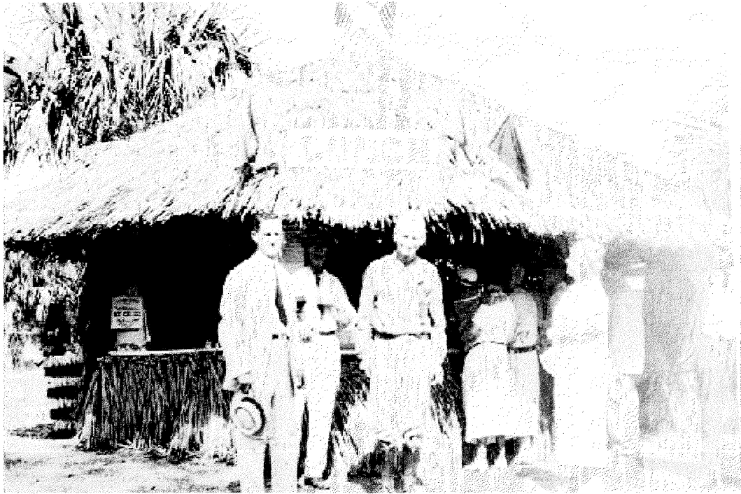
illustration 4.82 Rustic Tea Garden - thatched structure (Koreshan State Historic Site) The sign on the roof of this building reads "LUNCH."
