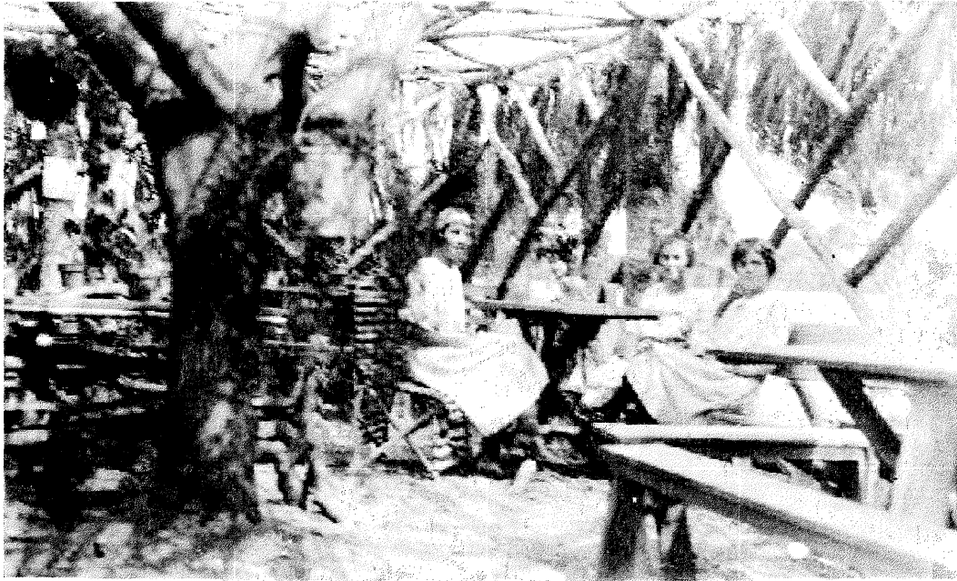
illustration 4.86 Rustic Tea Garden - Rustic Trellis House (Koreshan State Historic Site) In this photograph, rustic chairs and tables can be seen inside the trellis structure, as well as a tree which seems to be growing inside.
