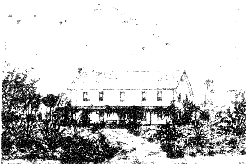
illustration 4.15 Edith Campbell drawing of the Founder's House shown from the north (Herbert-Reeves, p. 58) In this view of the north side of the Founder's House, the porch is visible, which appears to be planted with vines. Along the walkway can be seen row of small agave-like plants.
