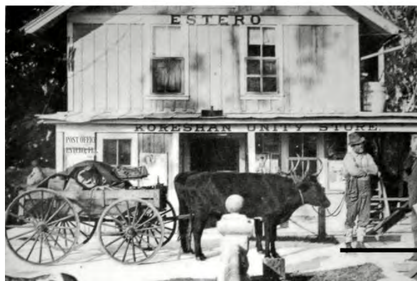
Estero Post Office and General Store
